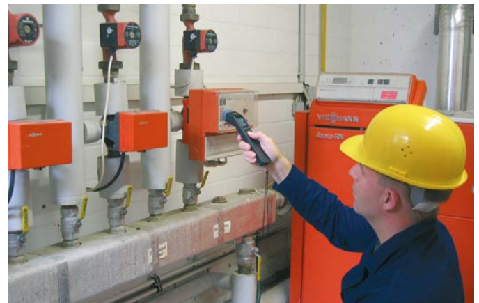
Temperature monitoring of heating circuits
